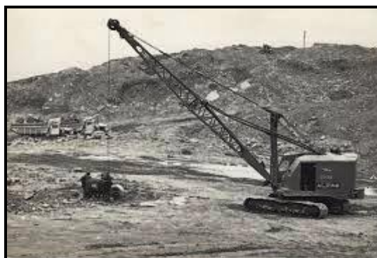
Figure 7 – 1970s quarrying, a Ruston dragline like those used at the Norman Works, operated largely by one person ( http://www.flickr.com )
