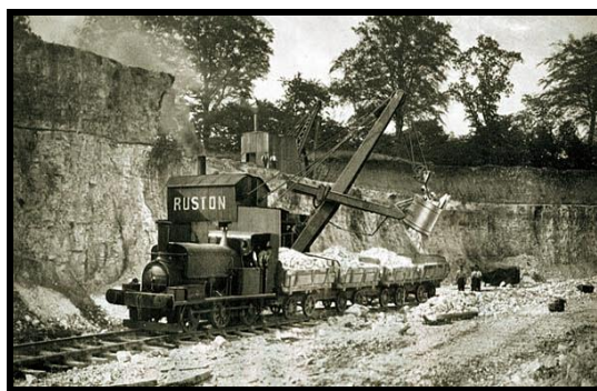
Figure 5 – early mechanised quarrying, straight onto rail transport ( http://www.cementkilns.co.uk/millsetc.html )
