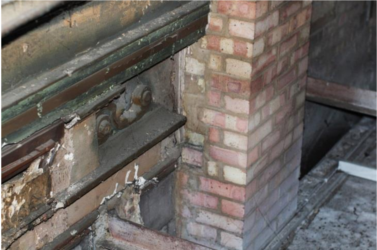
Figure 13 Playhouse alterations: reinforced pier [JIMG_1561]
