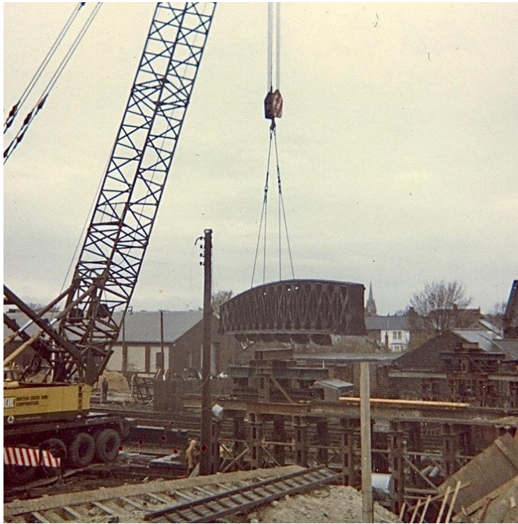
Figures 71 — Removal of the final side piece (photos: Barry Hurst: SO: 191-bh-bridge-demolition1d, 191-bh-bridge-demolition1c)
