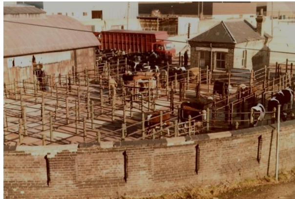
Figure 28 – Cambridge Cattle Market, showing cast iron posts and bars used to fence cattle. Many of these were made by J I Headly at Mill Road, 1880s.
