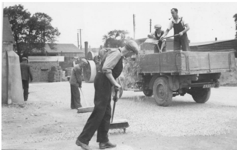
Figure 87 – Spreading granite chippings, 1936 (CC: B. Kings. K36.37181)
