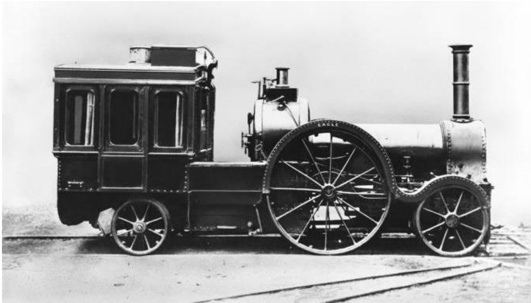
Figure 13 – The Eagle: the carriage was added later. See 'The Eagle' embossed on large wheel J & E Headly 1849 (National Rail Museum)
