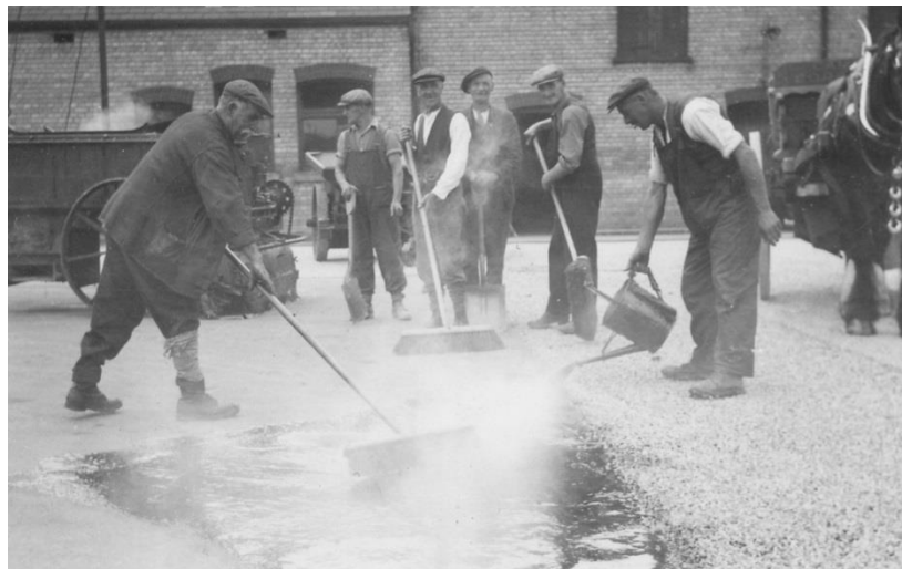
Figure 86 – Spreading tar, 1936 (CC: B. Kings. K36.37179)
