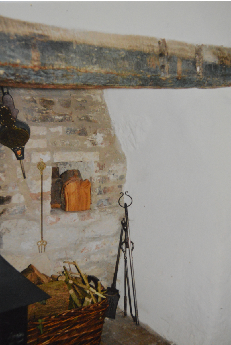
Photo 9. Corner of the smaller cleared inglenook at No. 44, showing salt recess and holes in the beams to support cooking pots and meat on spits.
