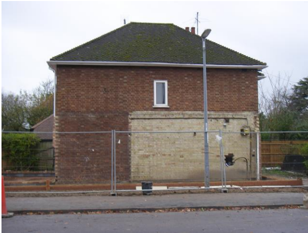
Fig 30: Demolished garage revealing the use of Gault bricks for internal wall construction, Queen Edith's Way c1930
