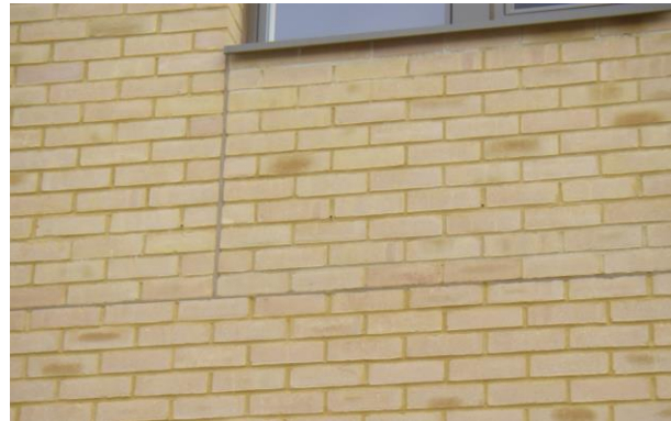
Fig 47: “Matching” bricks in stretcher bond – rain screen cladding over a steel frame
