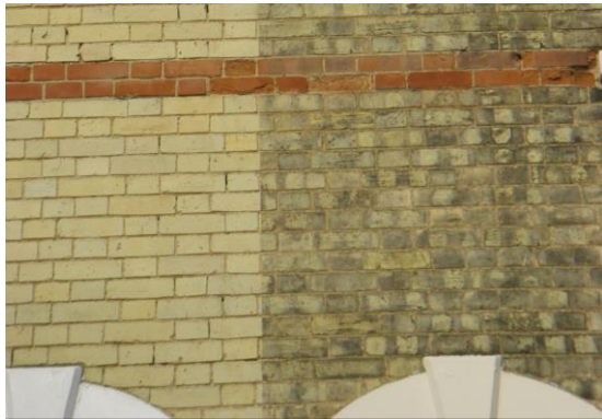
Fig 46: Clean & dirty “Gault bricks” in load bearing Flemish bond
