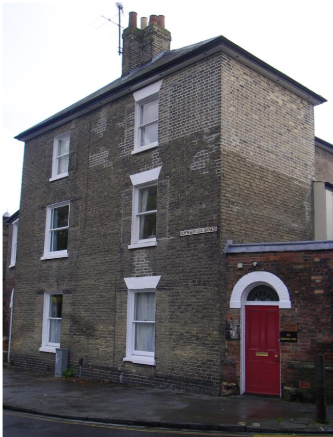
Fig 54 Undisguised repointing
