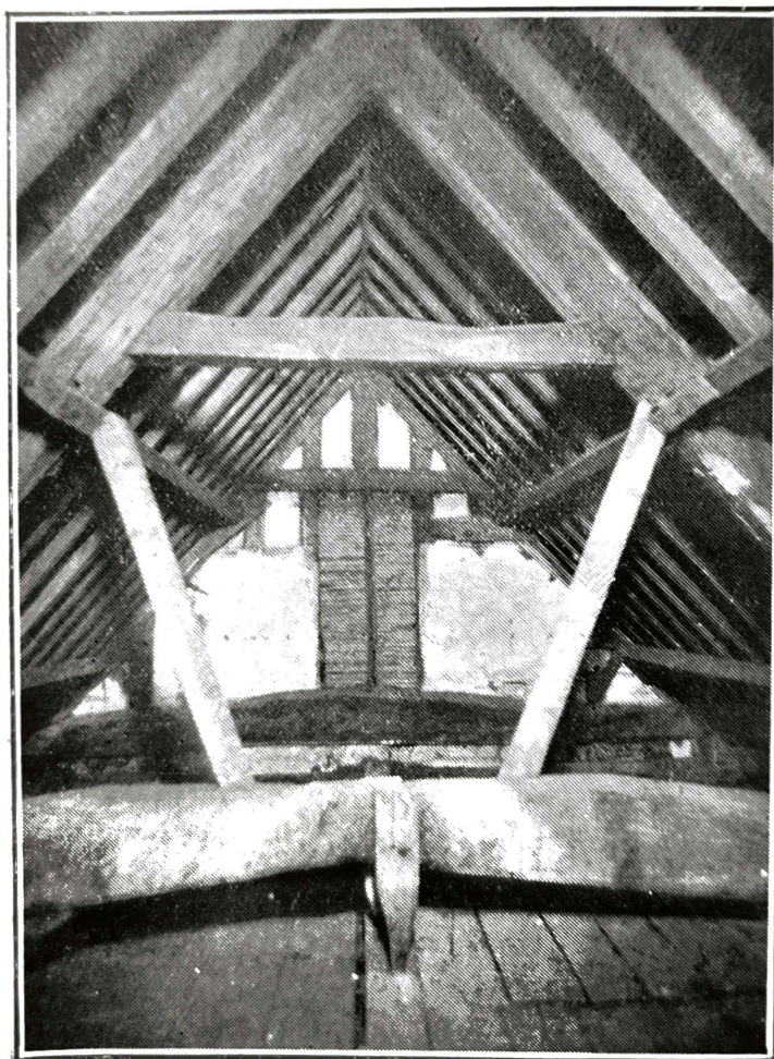
A view of the attic at Lordship Farm, showing a blocked up window. This was probably glazed when the roof was thatched and the room could be used as a cheese room. The end wall is made of clay laid on reeds.
