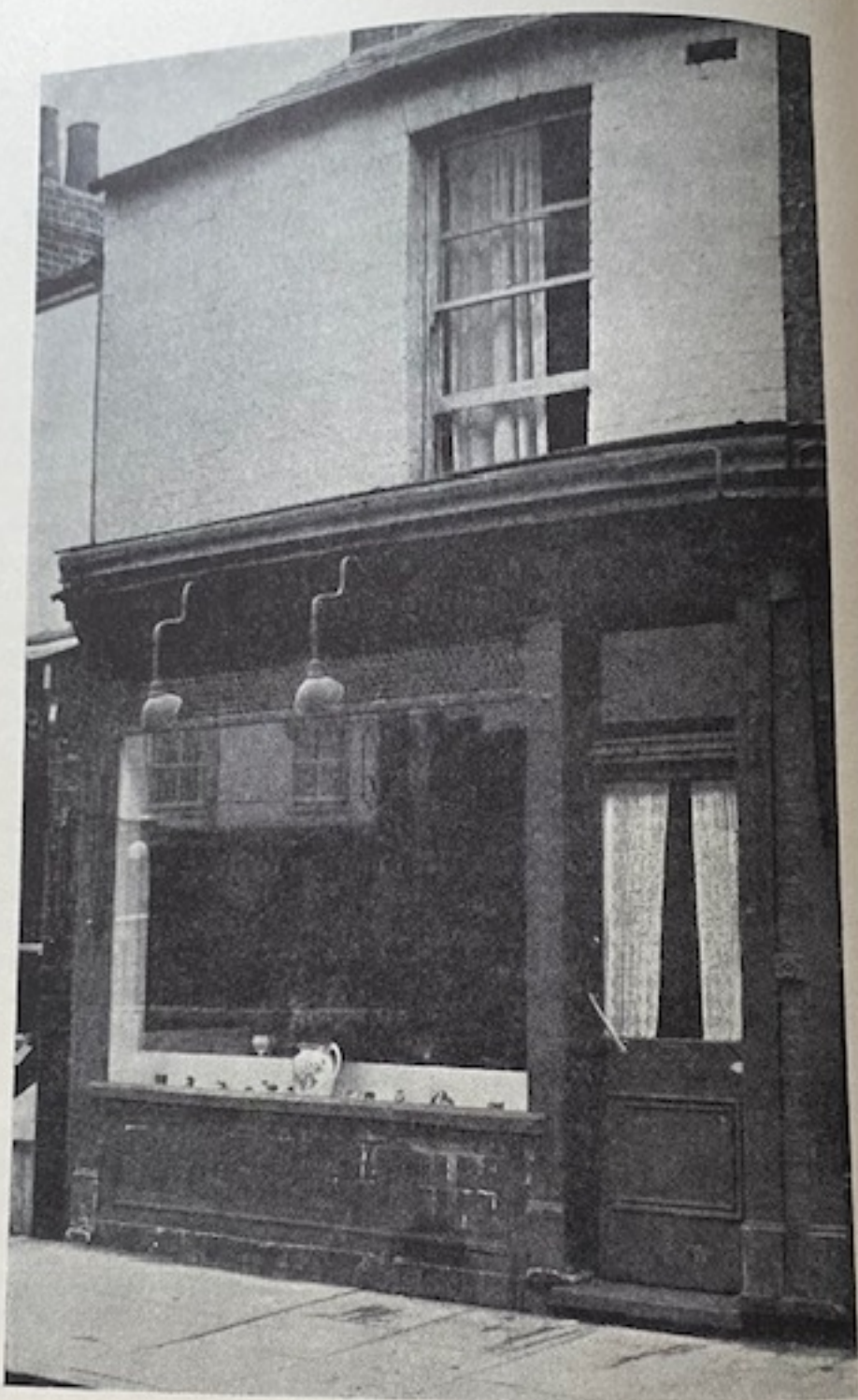
104, FITZROY STREET, 1876 The shop window has been modernised
