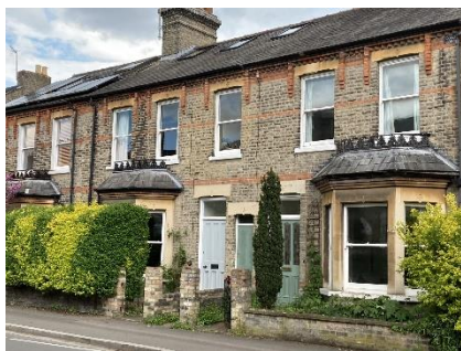
Figure 11 — red corbels and eaves (75–79 Tenison Road)
