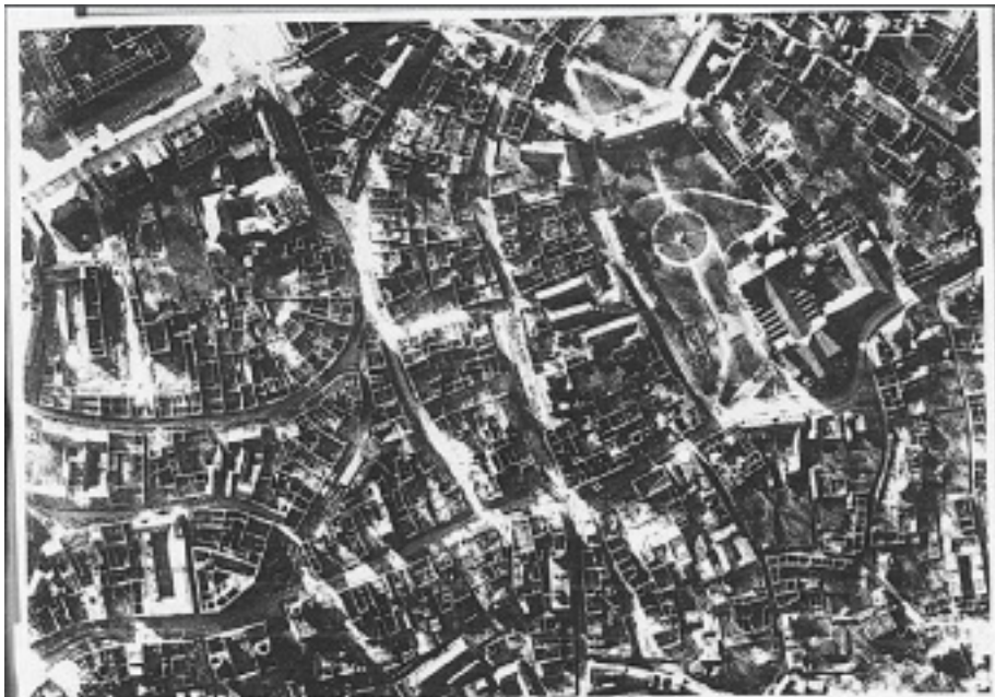
13.11 Photograph taken after the attack on 25th/26th February, 1944 shows the vicious destruction by fire in the commercial and administrative centre of the town.
