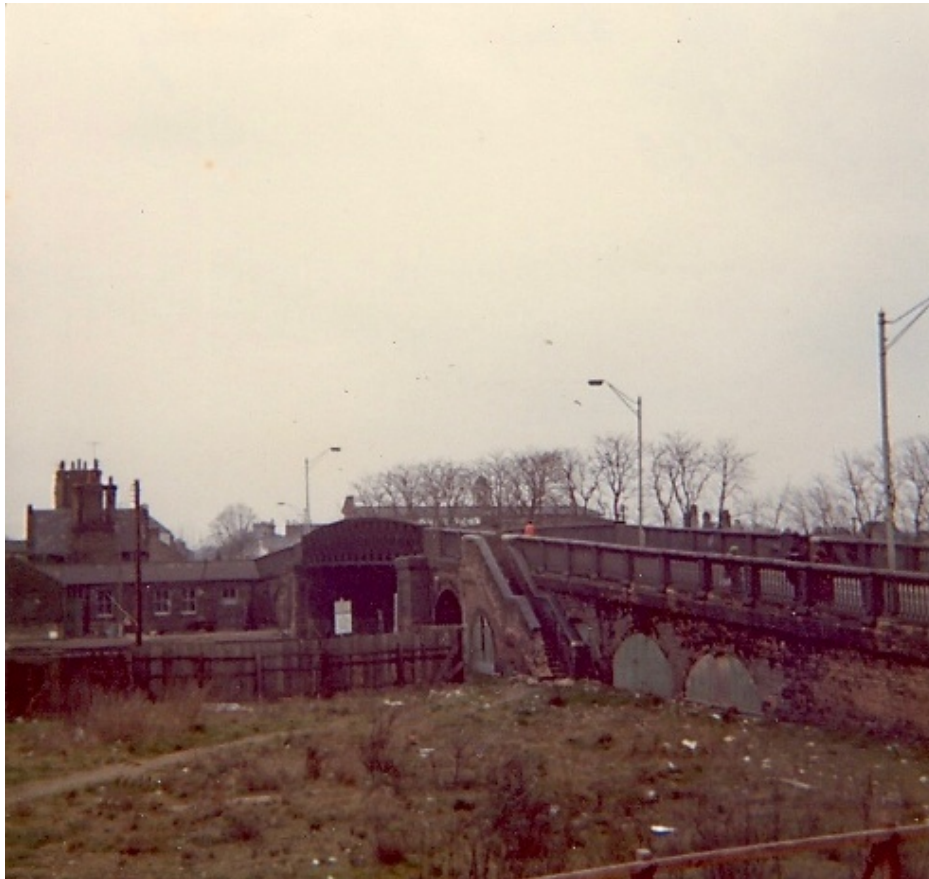
43. Mill Road bridge from Argyle Street, late 1970s. (MRHS. Courtesy of Barry Hurst)
