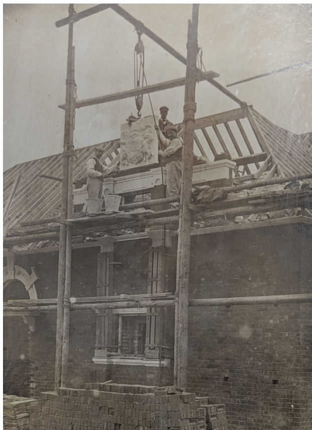
24. Romsey School under construction, 1905. (CA. C/ES20S/3/2/16)
