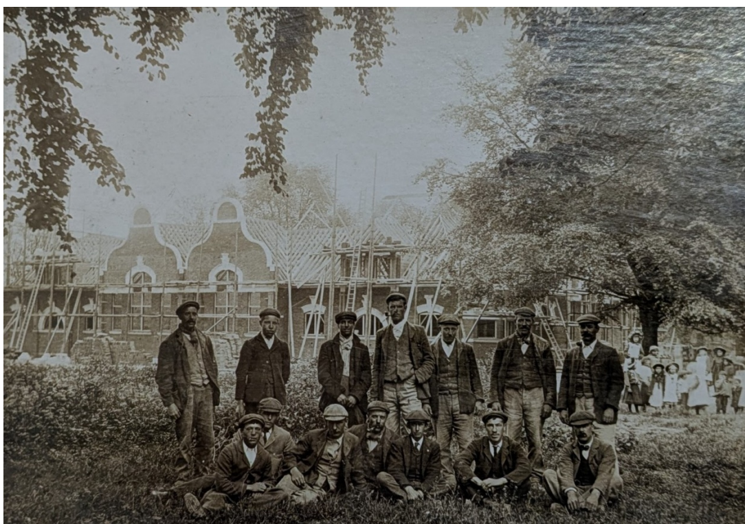
25. Romsey School under construction, 1905. (CA. C/ES20S/3/2/16)
