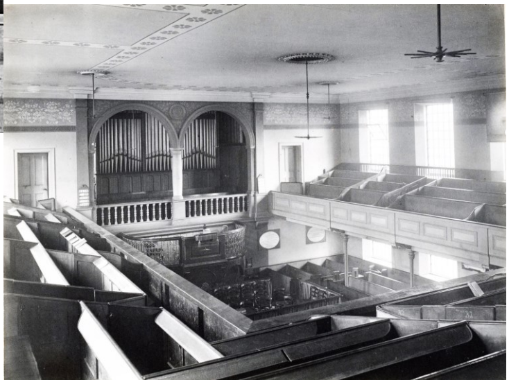
Fig. 17 St Andrews Baptist Chapel. 1855 Interior
